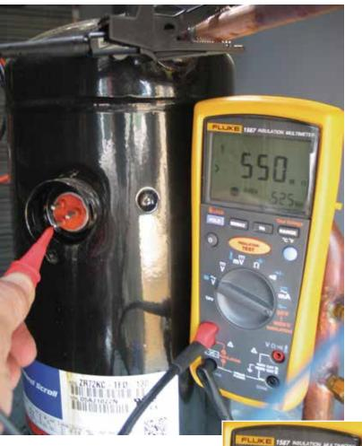
At an applied voltage of 500V, this IRT reading shows >550 M $\Omega$ , indicating resistance is out of range. A second IR test was performed at 1000 V and showed 1.1 G $\Omega$  (1100 M $\Omega$ ). If no leakage current had been detected, a reading would have been >2.2 G $\Omega$ . The Fluke 1587 insulation multimeter combines the features of a DMM (volts, ohms, millivolts, milliamps, frequency, capacitance, temperature) with a megohm meter for comprehensive motor maintenance.
